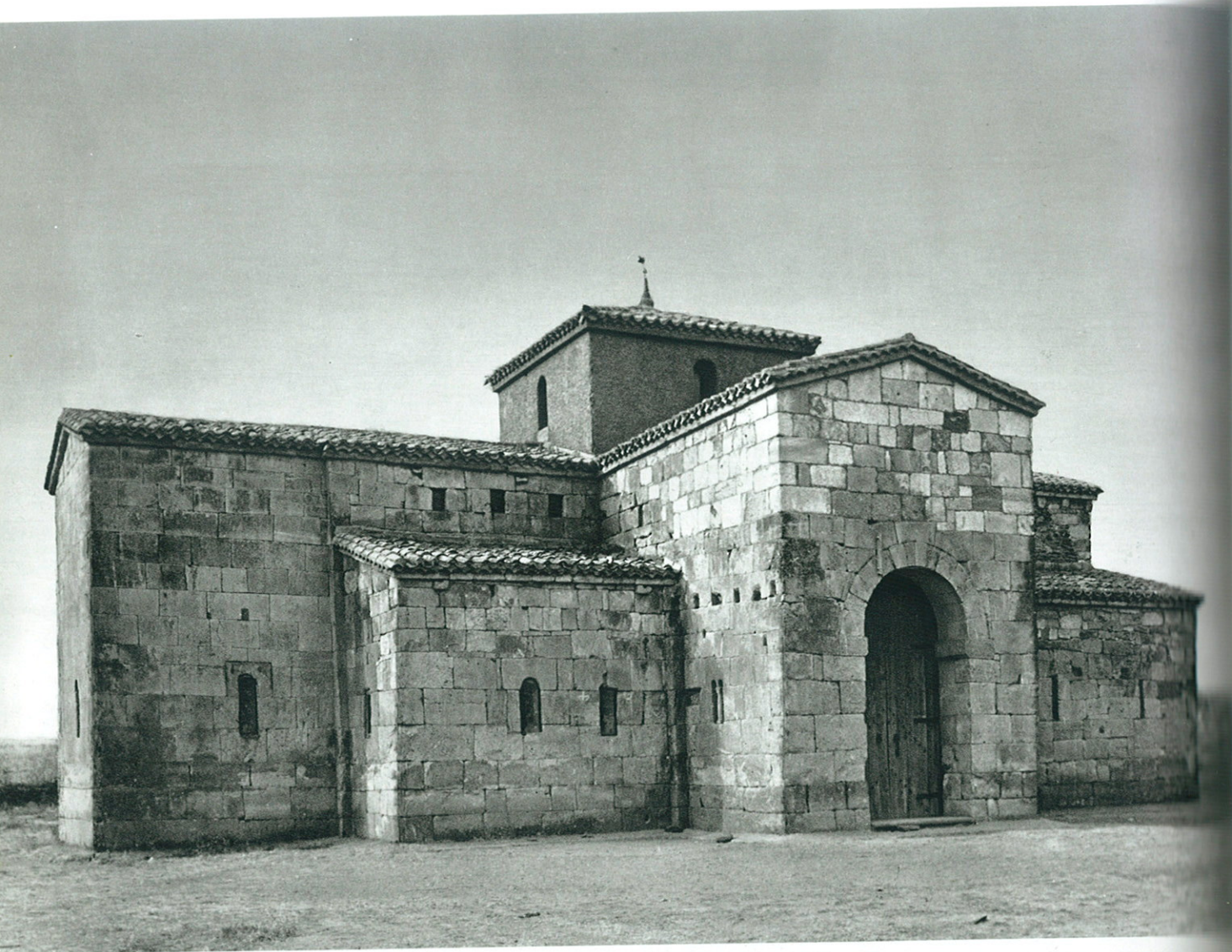
98 - SAN PEDRO DE LA NAVE. EXTERIOR FROM THE SOUTH-WEST.
